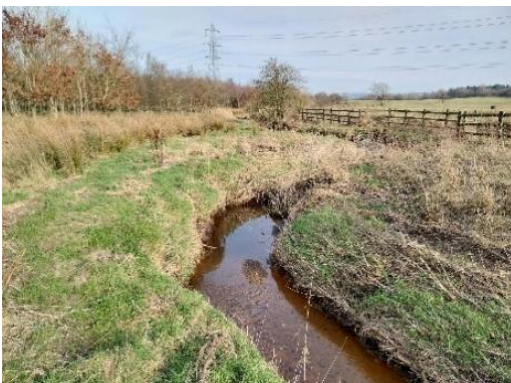
Figure 37 image showing the colour of the brook just after the motorway outfall. on the left-hand bank is the area for potential wetland
