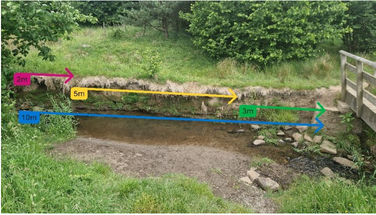
Figure 44 Suggested dimensions for cliff reprofiling
