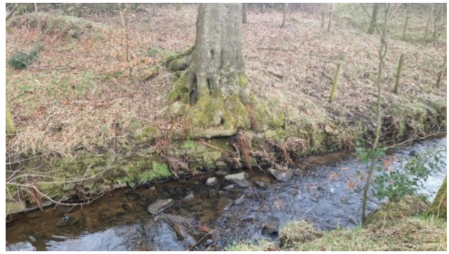
Figure 18 SD72340 27220, Example of revetment location where removal will not be viable.
