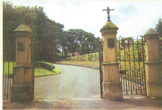
Oak Hill park gates on Manchester Road 19
